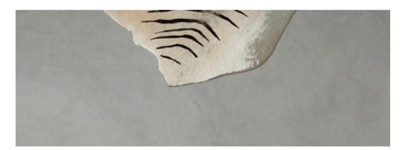
Apply a first coat and possibly a second coat of Morpheo M350 Ultra-Fin, in a thin layer. These finishing coats determine the final grain of the coating and allow it to be smoothed. These coats will be applied with a smoothing trowel in the direction of the coats of Morpheo M700 Classic or Morpheo M700F Fluide.
